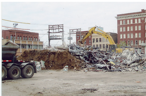
Demolition of the Lark Theatre/Cinema Grill in downtown Fargo makes room for the new Cityscapes Plaza.
