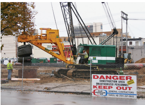
Caissons being drilled to a depth of 107 feet and filled with concrete.
