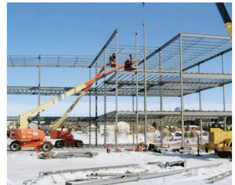
The three-story primary steel structure being erected.
