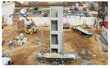
Above: An aerial view of the site, featuring the elevator shaft that will be in the center of the Mark Apartments. Right: Crews place the forms for the walls.
