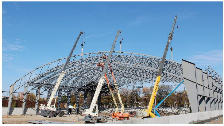
The curved roof taking shape at the UND Athletics High Performance Center on the campus of the University of North Dakota in Grand Forks. Below: Numerous cranes were required as the roof trusses are set.
